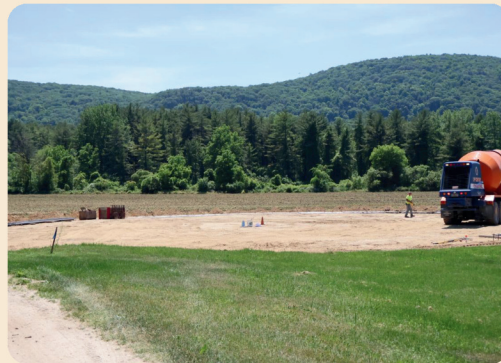
Leveling the Ground
