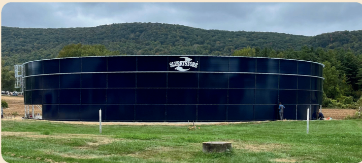
Finishing the Storage Tank (man for scale)
