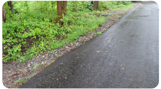
Sediment and gravel deposited on side of a local road after extreme rain event, draining into nearby stream
