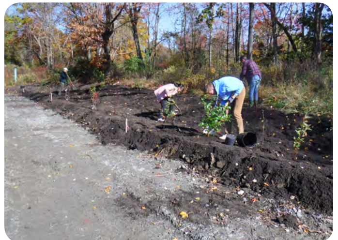
In the top picture is NWCD staff installing a rain garden behind the Bethlehem Town Hall. The bottom two pictures are Taft School volunteers planting a rain garden by the Heminway Municipal Office Building in Watertown
